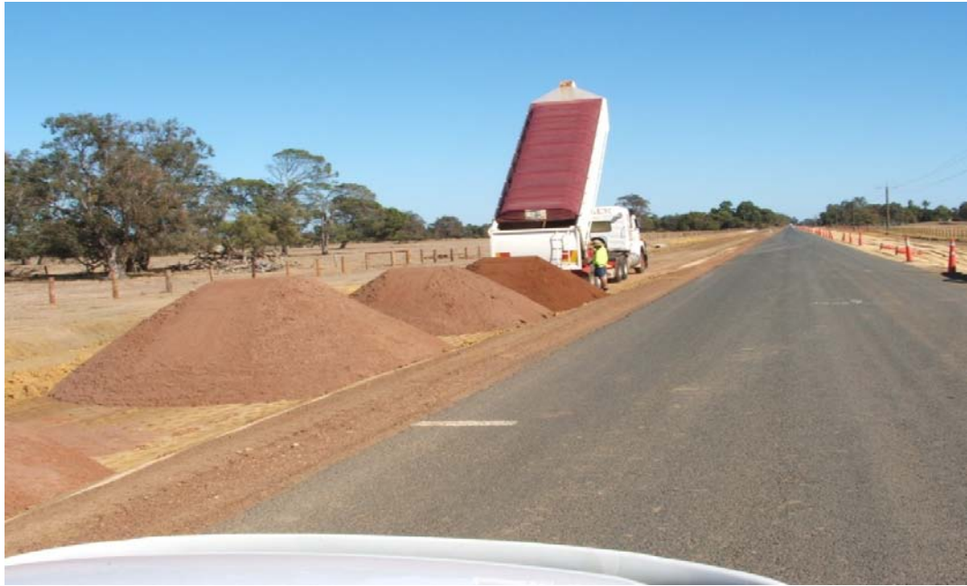
Figure 8 – Use of Red Sand™ for road construction (Photograph courtesy of Alcoa)
