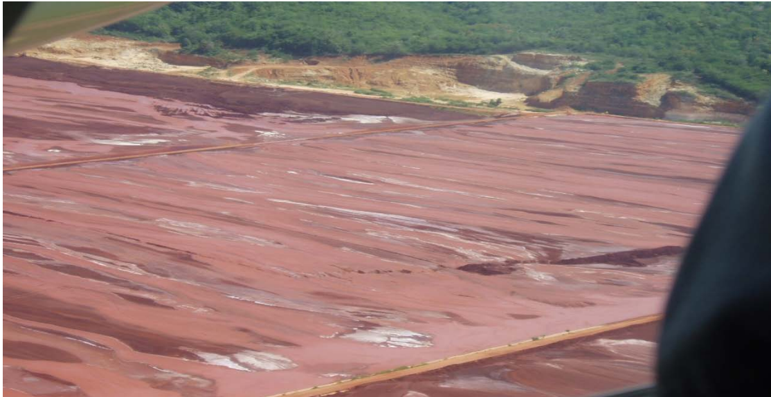
Figure 5 – Mud dewatering and compaction
